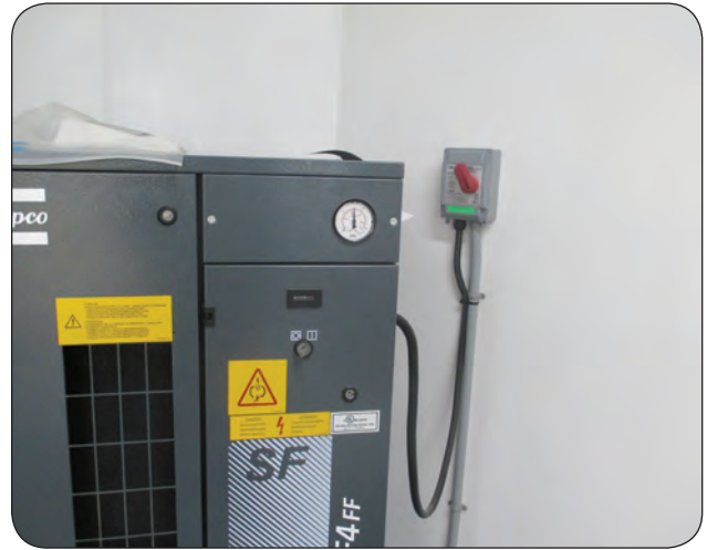
Figure 8. Hard-wired compressor.
