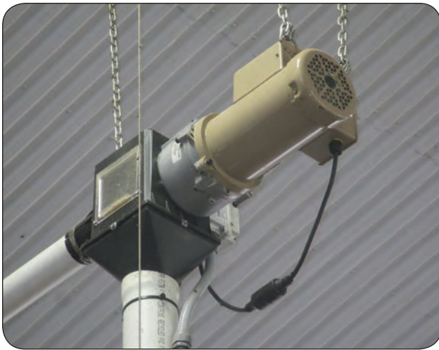
Figure 9. Wet-rated plugs and receptacles with hard-wired cables are recommended for use in barn environments. Source: Heartland Farm Mutual, Waterloo, Ontario.
