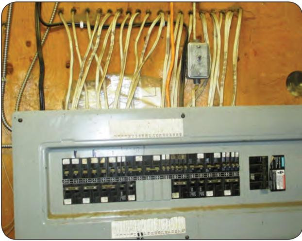
**Figure 6.** Recessed wiring.
