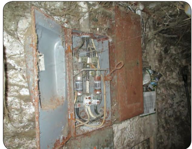
**Figure 4.** Corroded disconnect panel.
