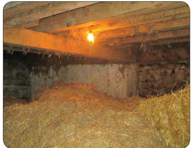
**Figure 13.** Flammable material near light fixture.
