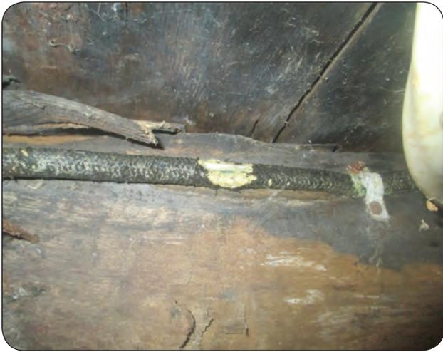
**Figure 5.** Rodent damage on electrical cable.
