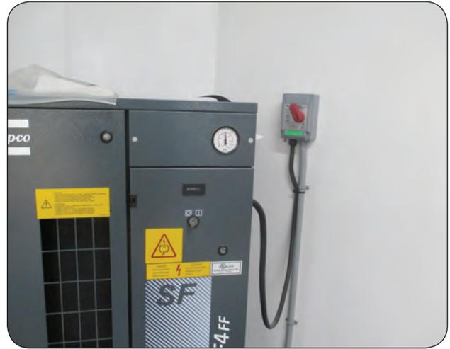
**Figure 8.** Hard-wired compressor.
